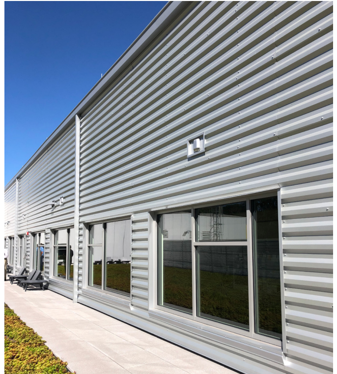
Photo D: Series MOE exterior wall packs, which were inset into ribbed exterior wall panels, using custom recessed tray.
