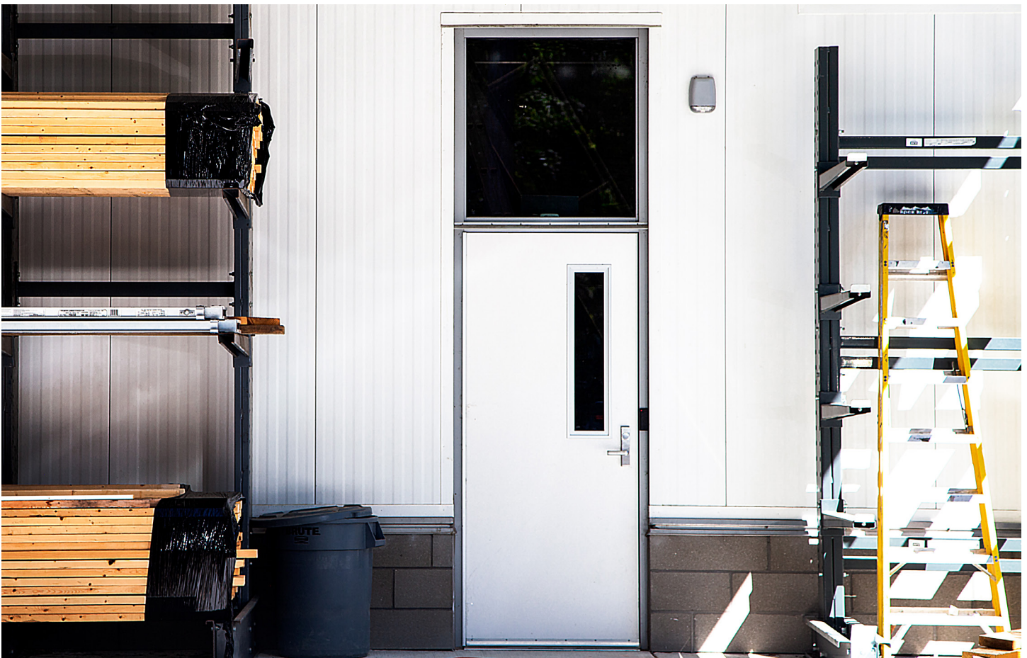
Photo E: Series MOE exterior wall packs mounted outside shop classroom door.
